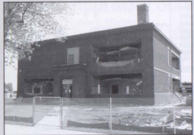
The demolition begins ...
